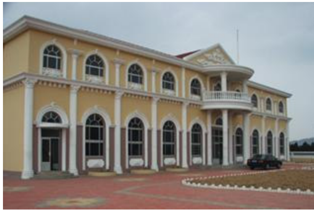
The facility building at the SWRO plant in Changdao, China
